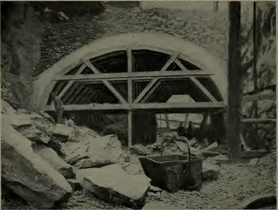
Concrete Arch Subway Construction in Open Cut.
